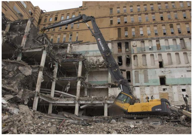
Volvo EC700C HR High Reach Demolition Excavator
